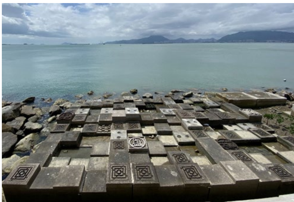
Example: Eco-shoreline at Tung Chung (bio-blocks)
